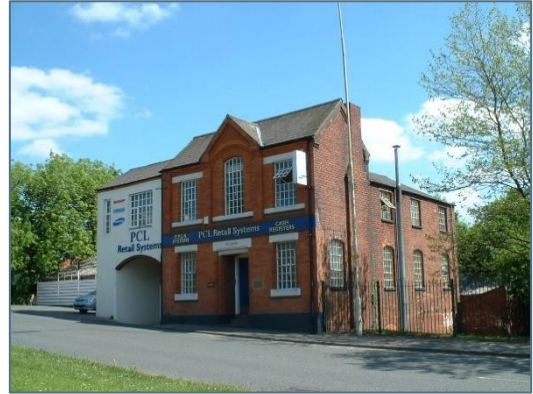
Mucklow Hill Offices Dudley © Dudley MBC
