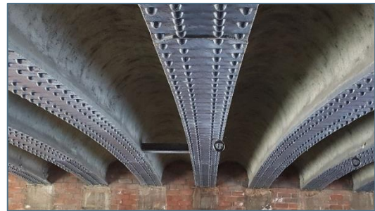
Horsley Fields Bridge detail
